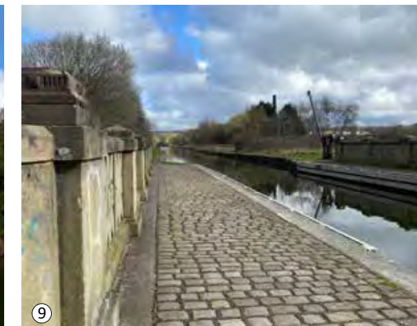
9 Grade II listed Aqueduct along the 'Straight Mile', Burnley
