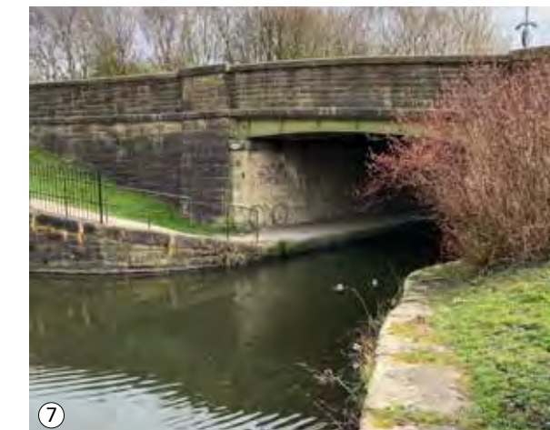
7 Bridge near Enfield Wharf, Hyndburn
