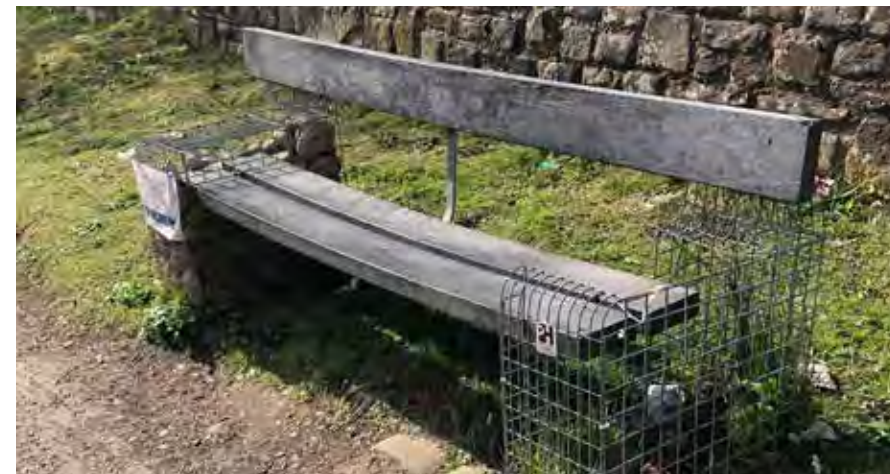
Damaged seating areas surrounded by litter, Blackburn
