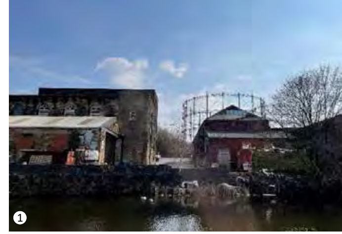
1 Brierfield Gasholder, Pendle
