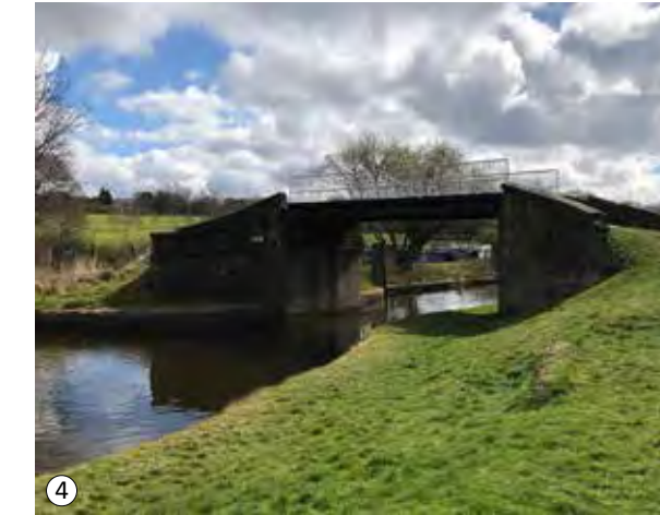
4 Bridge near Reedley Marina, Pendle
