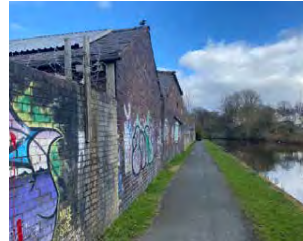
Industrial buildings backing onto the canal, Burnley
