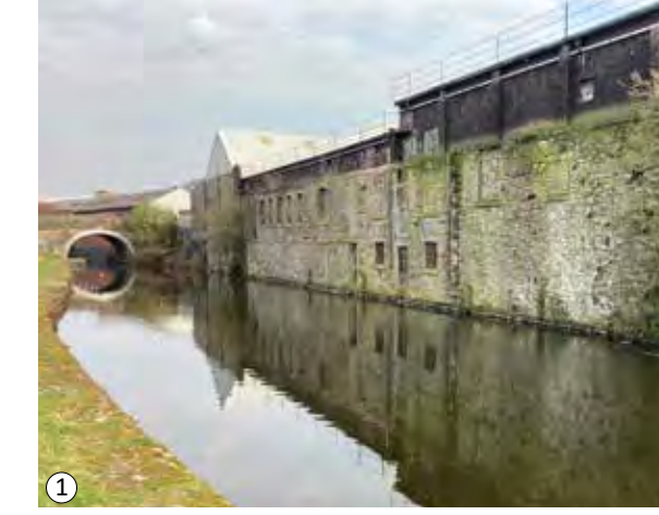
1 Facades/ Walls near Blackburn Station
