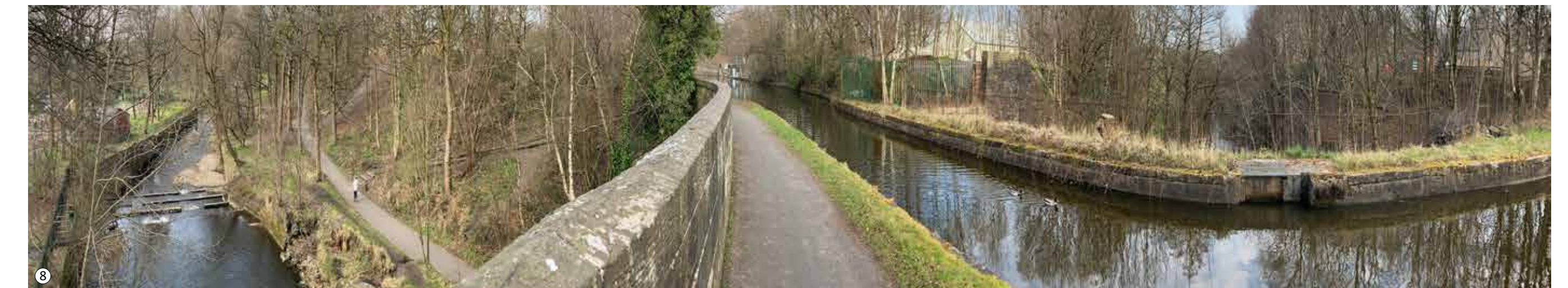
View from the bridge over Thompson Park, Burnley
