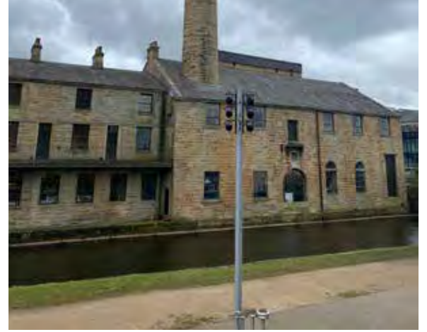
Lighting installation adjacent to Trafalgar Mill, Burnley
