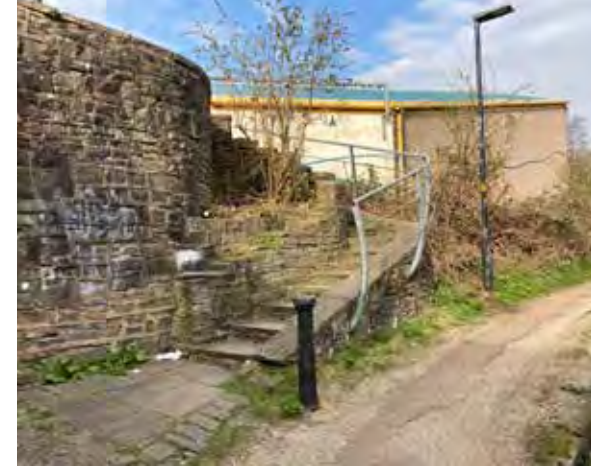
Low level lighting columns adjacent to bridges, Blackburn
