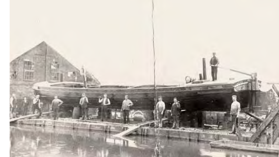
Construction of a canal barge: Blackburn with Darwen Library & Information Service: www.cottontown.org
