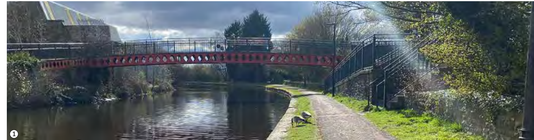
View towards pedestrian bridge near Blackburn Station
