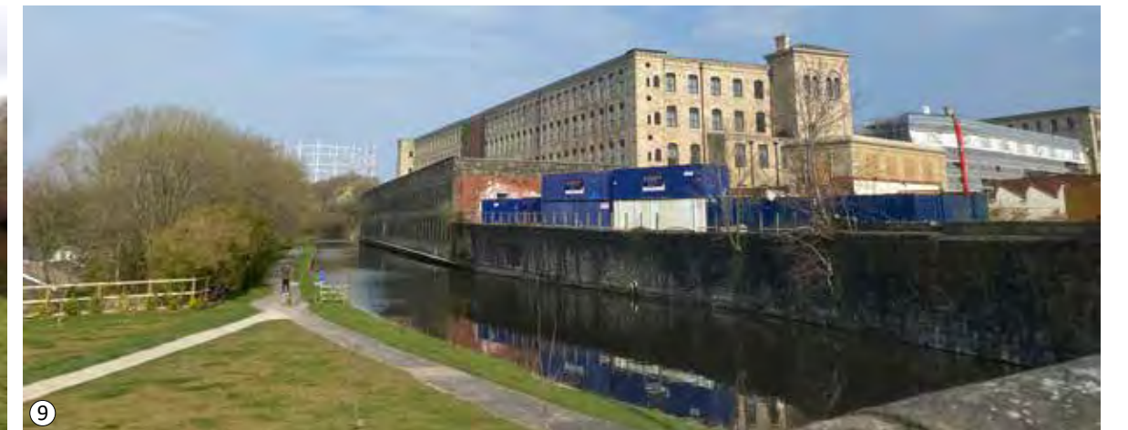
9 View from the bridge crossing towards Northlight, Brierfield
