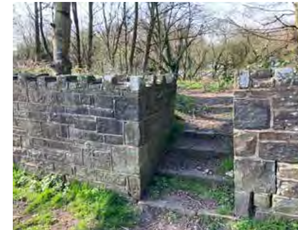
Stepped access to Thompson Park, Burnley
