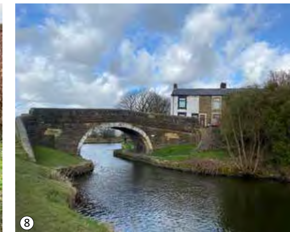
8 Grade II listed bridge, Church Kirk Bridge, Hyndburn
