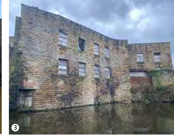
3 Derelict warehouse near Finsley Gate Wharf, Burnley
