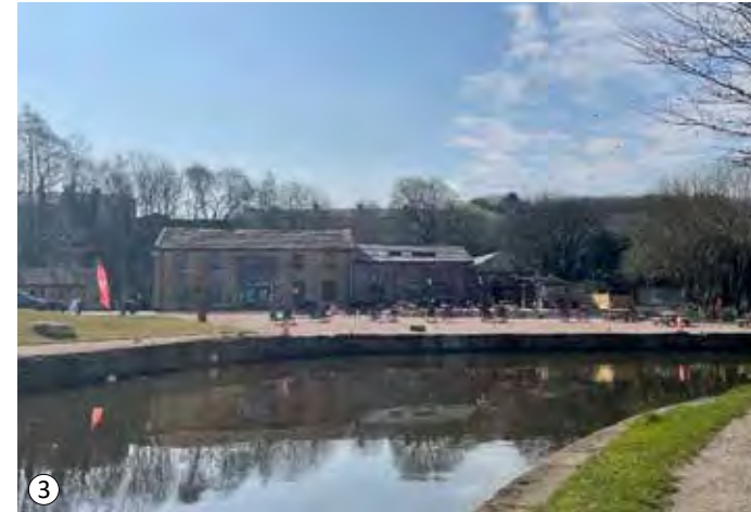
3 Grade II listed Finsley Wharf, Burnley
