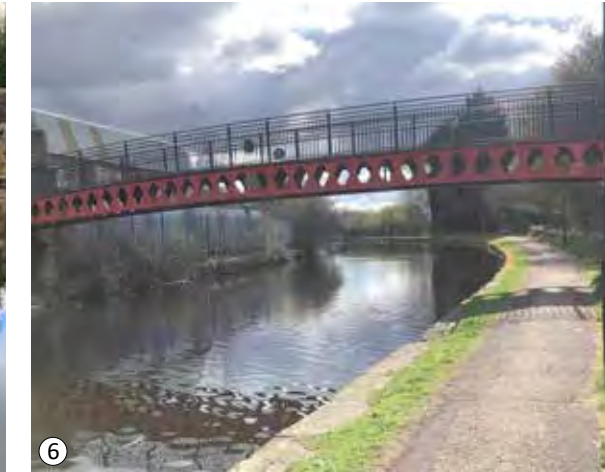
6 Bridge near Blackburn Station
